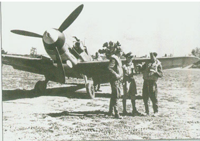
A Bf 109F-4/trop from I./JG 3 during operations in the Mediterranean in 1942. The aircraft is fitted with armoured glass and an under-fuselage carrier for a 250-kg bomb. (CAW)
