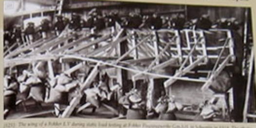
(121) The wing of a Fokker E.V. during static load testing at Fokker Flugzeugwerke GmbH, in Schweinfurt in 1918. The photograph shows its under surface with the characteristic diagonal streaks of paint, resulting from uneven coating of the ground with touch-applied stain. Note the camouflage colour division line to the left of the cross, between the darker Azur Violet and lighter Azur Blau.
